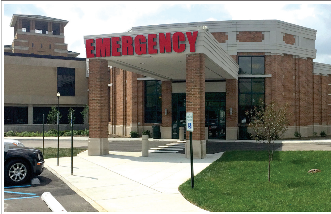
Today's main entrance to the Emergency Department. The new, larger department opened in 2016.
