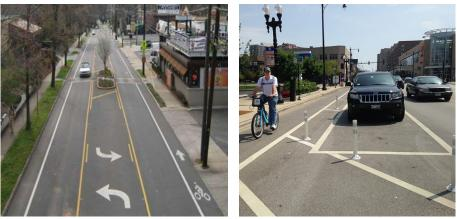
**Above:** Move the paint to create 10 foot travel lanes, which allows the additional pavement to be reallocated for other uses, such as parking and bike lanes, as seen in downtown Charlotte, NC (left) and Chicago, IL (right).
