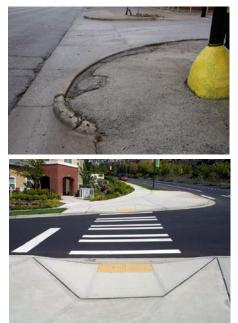
The corner pictured above (top) has an incomplete sidewalk and no curb ramp, forcing some pedestrians to go around, either onto a busy street, or into a parking lot in order to cross the intersection. The other corner pictured above (bottom) with curb ramps and crosswalk is much more safe and accessible.
